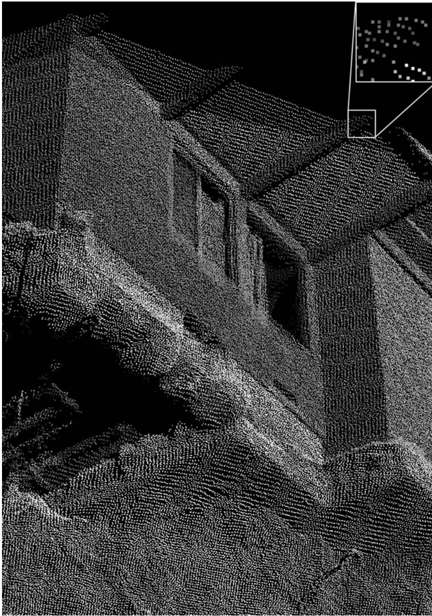
Fig. 1. A T-LiDAR scan looking up through the floorboards of a house after a landslide removed part of its foundation. The inset shows a close-up of the placard-based visualization, revealing gaps between reflections. (© Michael Neff)
